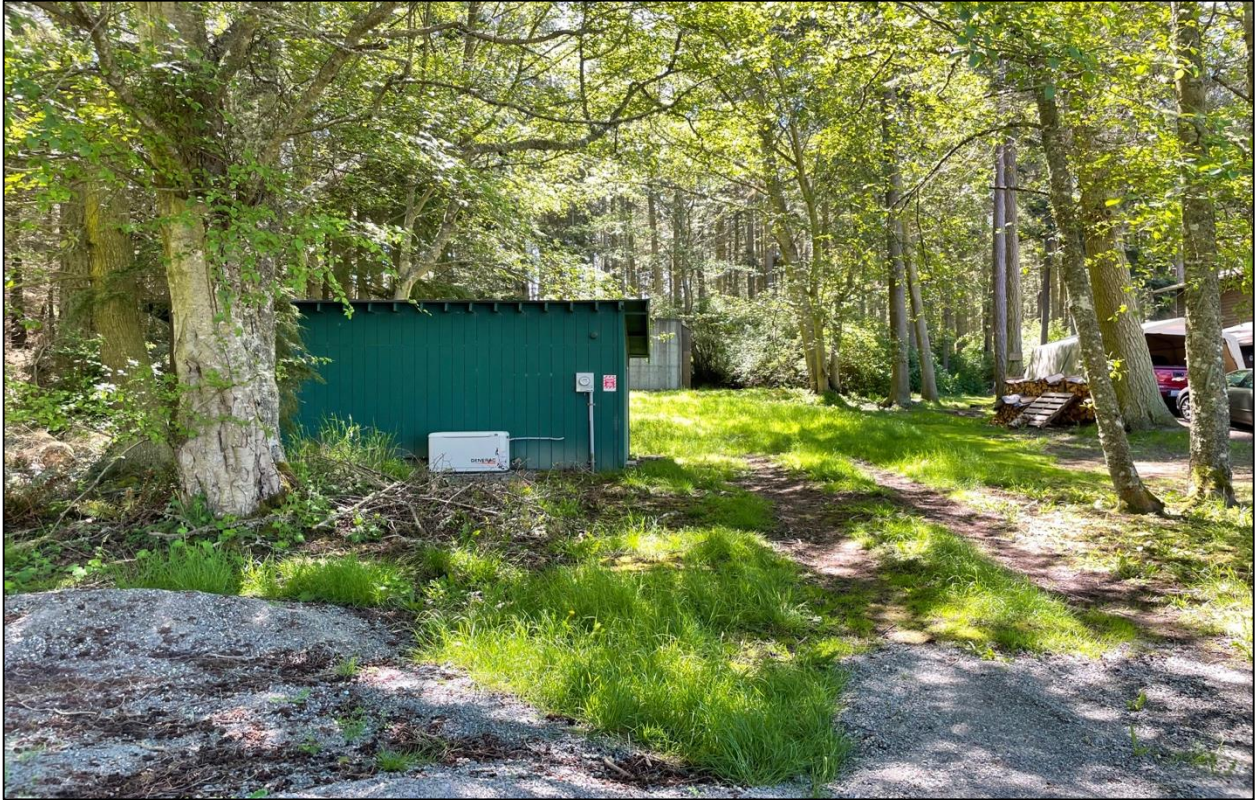
Photo 2. Southern view of the well located at 1957 West Even Down Way.
